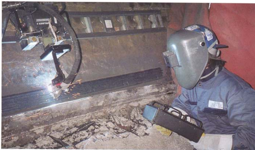
Fig. 4 — An optional gun axial slide bracket, combined with wide stroke steering, minimized the need for repositioning tracks.
