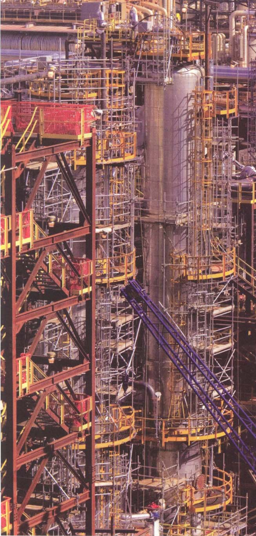
Fig. 1 — The cylindrical tower of a typical coker.
